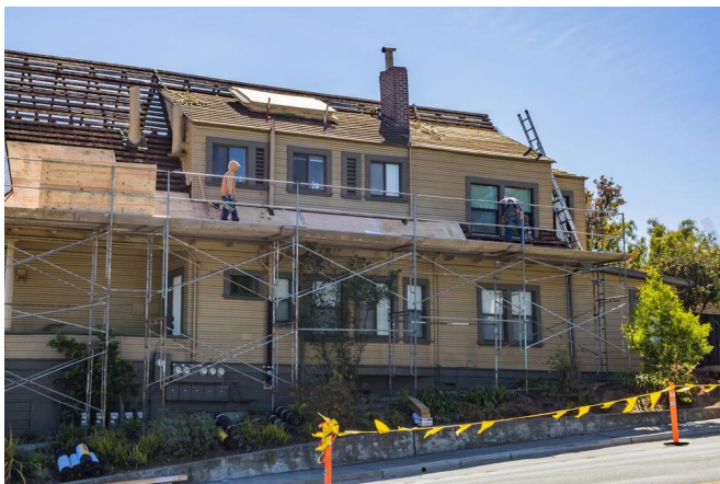
RP-1 A house under renovation, wrapped in scaffolding while the roof is worked on. Representative of the building type; not this property.
