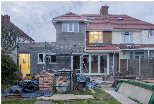
RP-2 A house in the middle of a major renovation, with a new rear extension under construction. Representative of the building type; not this property.
