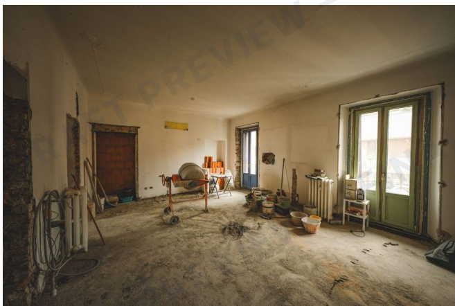
RP-3 An interior room stripped back during renovation, with bare walls and materials on the floor. Representative of the building type; not this property.
