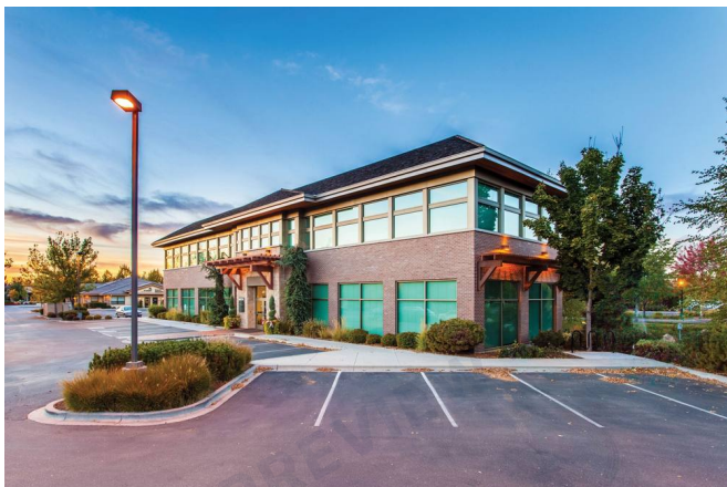
RP-1 A two story professional office building of the kind medical practices occupy, with surface parking. Representative of the building type; not this property.
