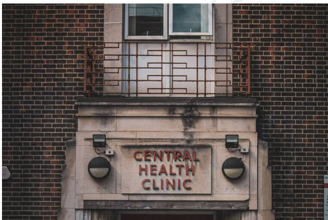
RP-3 The upper facade of a masonry health clinic, with the clinic name carved into the stone. Representative of the building type; not this property.
