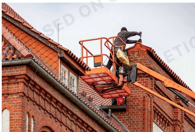
RP-2 Roof work underway on an older masonry building, carried out from a lift. Representative of the building type; not this property.
