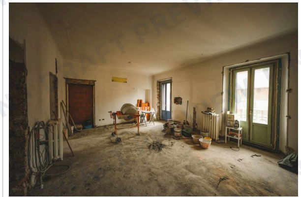
RP-3 An interior room stripped back during a unit renovation, with bare walls and materials on the floor. Representative of the building type; not this property.
