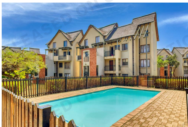
RP-2 Three story garden apartment buildings around a pool deck, a common amenity at complexes of this size. Representative of the building type; not this property.
